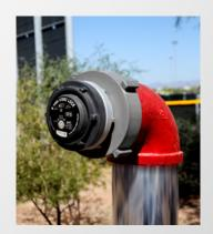
Knox Storz Lock secured onto a large FDC
